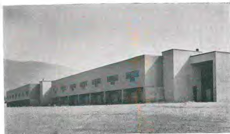
Area Vocational School under construction at Woodstock Avenue.
